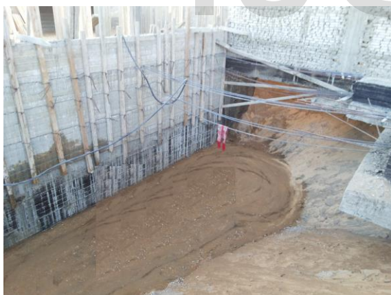
Fig. 2. Compacted replaced soil (non-retaining the adjacent Neighbour structures)
